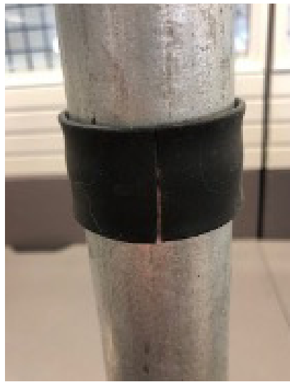
FIGURE 19: Seal on Pipe
