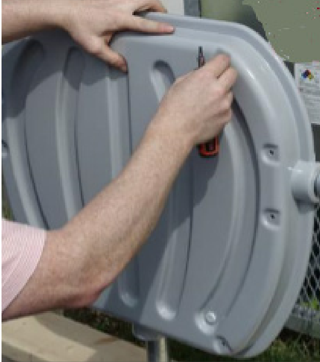
FIGURE 23: Plastic Shell Install
