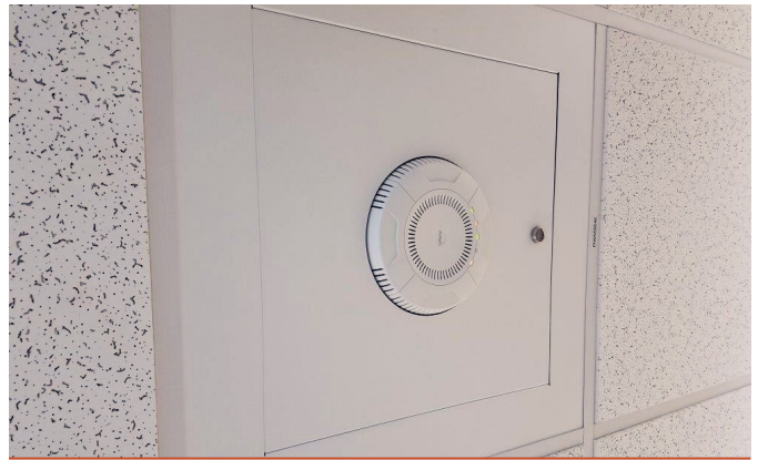
Ceiling Tile Enclosures for Access Points
